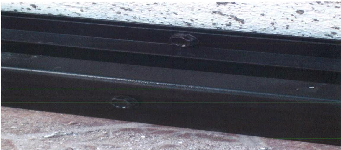
Below: Walkover track. Must use flat headed tapcons so they do not interfere with bushings when closing shutter. If making removable you must use the round head truss bolts.
