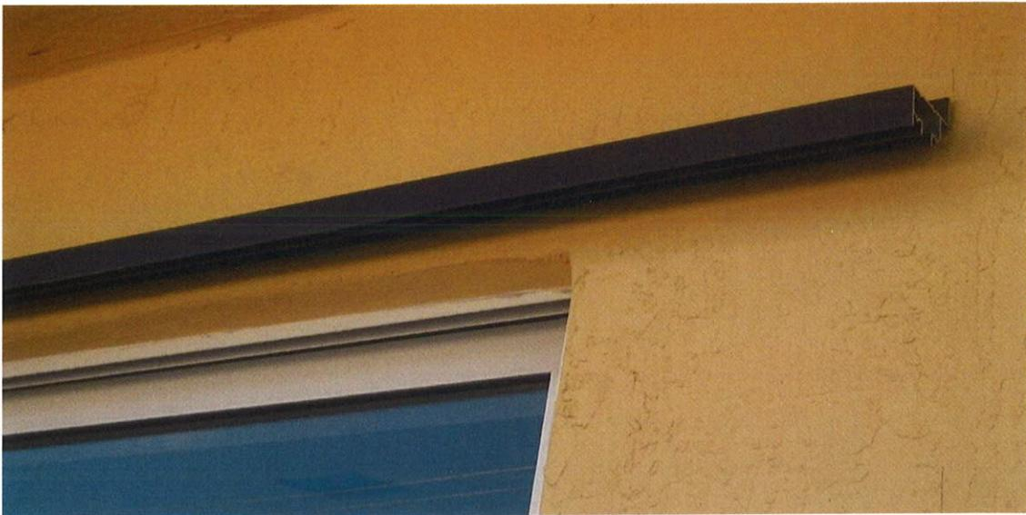
3.) Install one side angle and level from the end of the top track.
