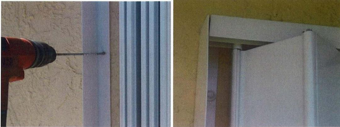
6) Make sure accordion stack is completely open and tightly stacked before attaching the accordion starter to the angle with #10 x 3/4 tech screws.
